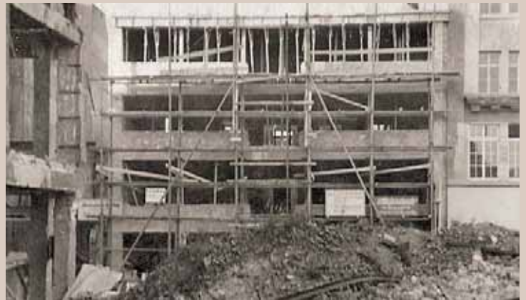
The new store before the reconstruction.
