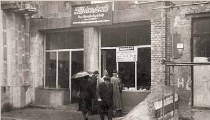
Provisional store during the reconstruction.
